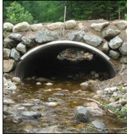
Figure 9. Before and after photos of a culvert replaced with a fish-friendly culvert ( California Fish Passage Forum ).
