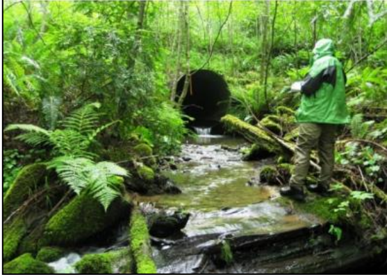
Figure 11. Before and after photos of a culvert replaced with a bridge ( California Fish Passage Forum ).
