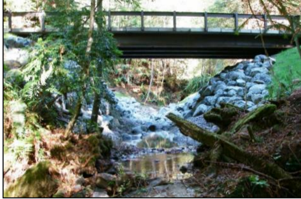
Figure 11. Before and after photos of a culvert replaced with a bridge ( California Fish Passage Forum ).
