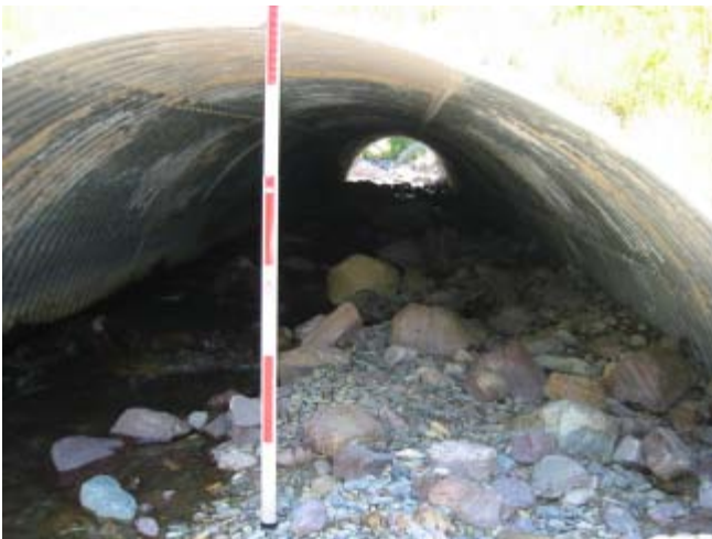
Riverside Creek 8/25/03 Looking upstream at culvert outlet.
