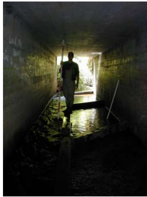
Adobe St Bridge on San Pedro Creek 5/28/03 In culvert looking upstream.
