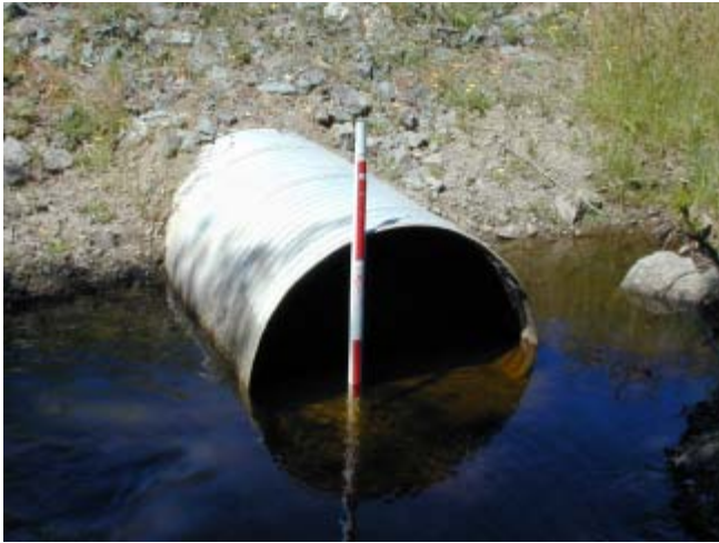
Merriman Creek 7/10/03 Looking upstream at culvert outlet.
