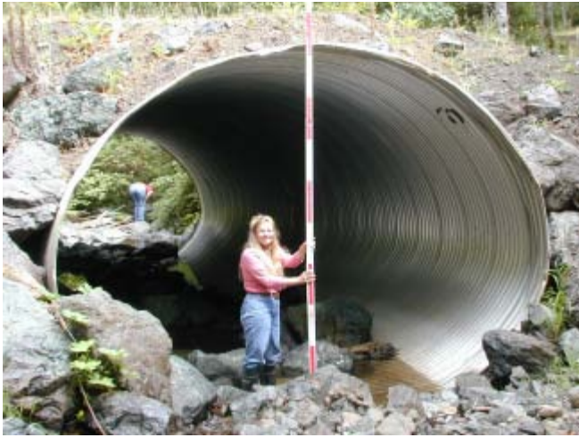
Indian Creek 7/10/03 Looking downstream at inlet of culvert.
