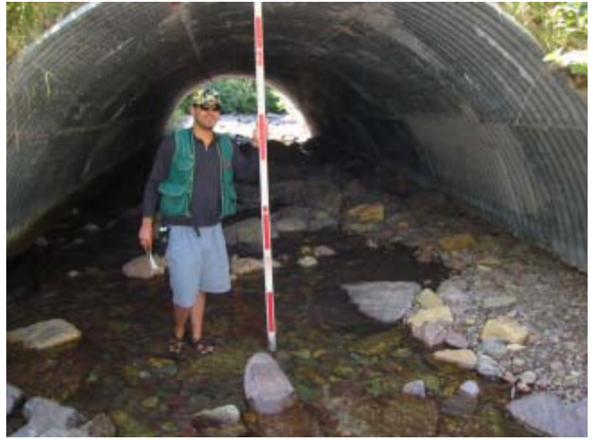
Margaret Creek 8/25/03 Looking downstream at culvert inlet.
