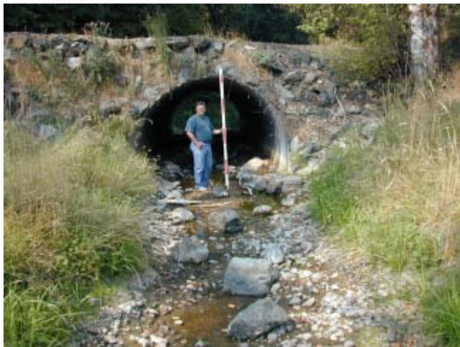
Green Creek 9/ 2/03 Looking upstream at culvert outlet.
