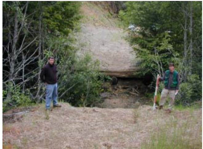
Little North Fork Navarro 5/30/03 Decommissioned road-stream crossing, Jamie Glasgow with Chris Surfleet, hydrologist for Mendocino Redwood Company.
