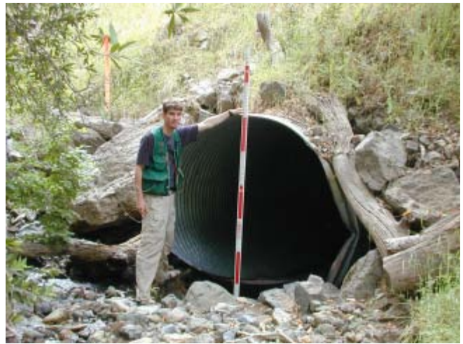
Feliz Creek Watershed 5/29/03 Looking downstream at culvert inlet.
