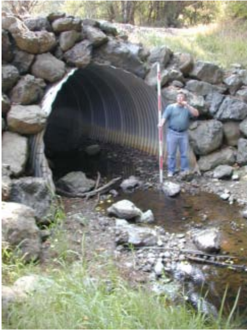
Green Creek 9/ 2/03 Looking downstream at culvert inlet.
