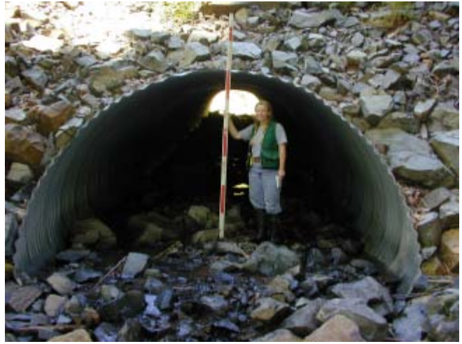
Finn Creek 7/ 9/03 Looking upstream at culvert outlet.
