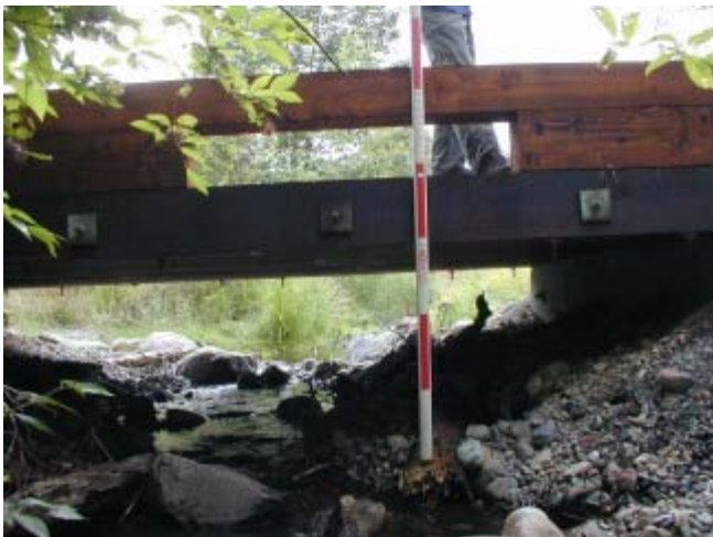
North Fork Newaukum Creek 8/11/03 Looking upstream at bridge, lower site.
