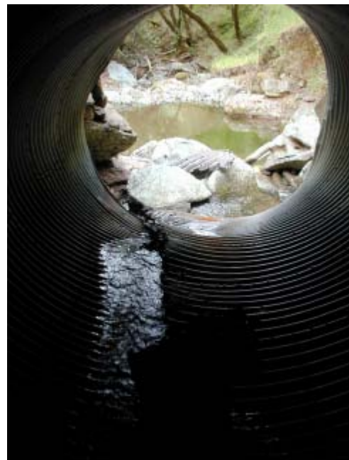
Feliz Creek Watershed 5/29/03 In culvert looking downstream.
