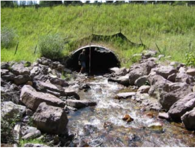
Harris Creek 8/25/03 Looking downstream at culvert inlet.
