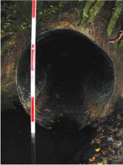
Hantz Creek 7/14/03 Looking upstream at culvert outlet.
