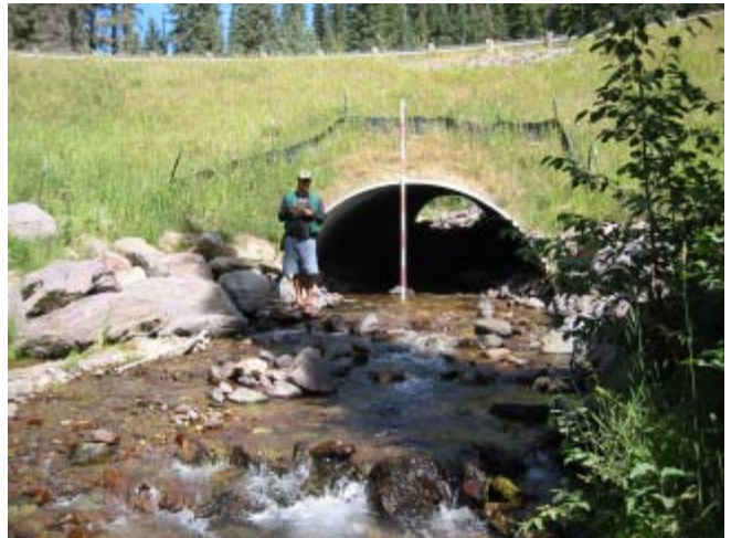
Harris Creek 8/25/03 Looking upstream at culvert outlet.
