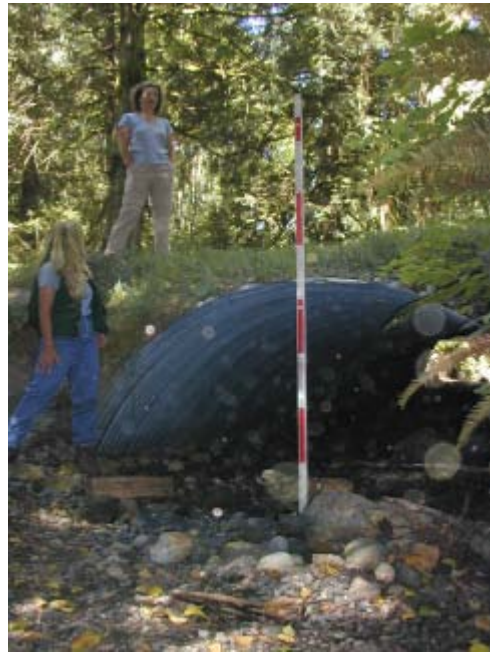
Klahoya Creek 8/18/03 Looking upstream at culvert, MaryLou White and Alison Studly.
