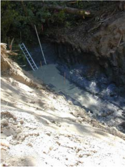
Shoeshel Creek 8/18/03 Creek downstream of the excavator work.
