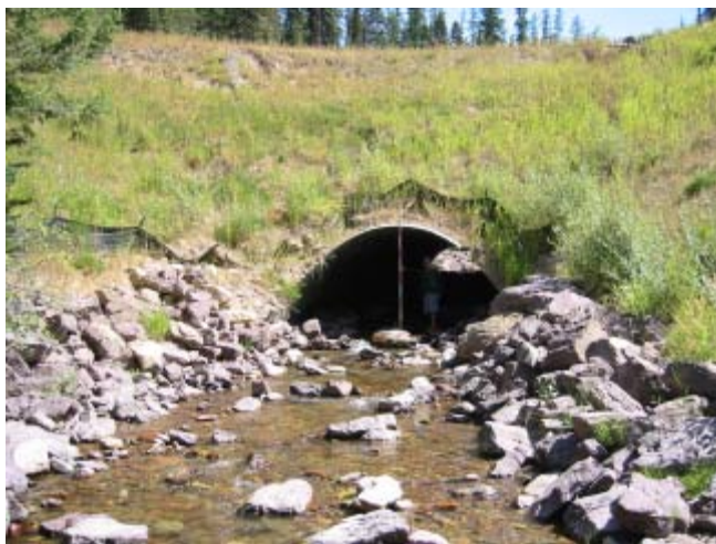
Felix Creek 8/25/03 Looking upstream at culvert outlet.
