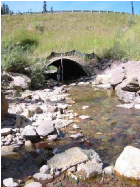
Felix Creek 8/25/03 Looking downstream at culvert inlet.
