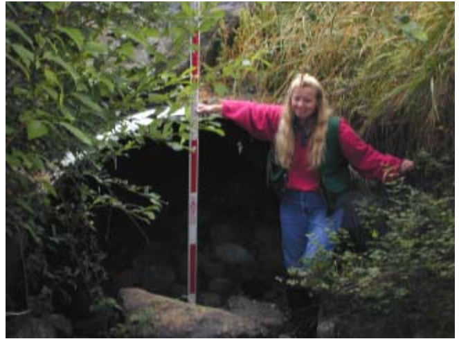
Edson Creek 7/10/03 Looking downstream at culvert inlet.
