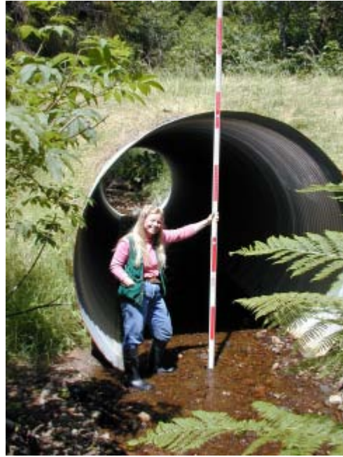
Hubbard Creek 7/10/03 Looking upstream at outlet.
