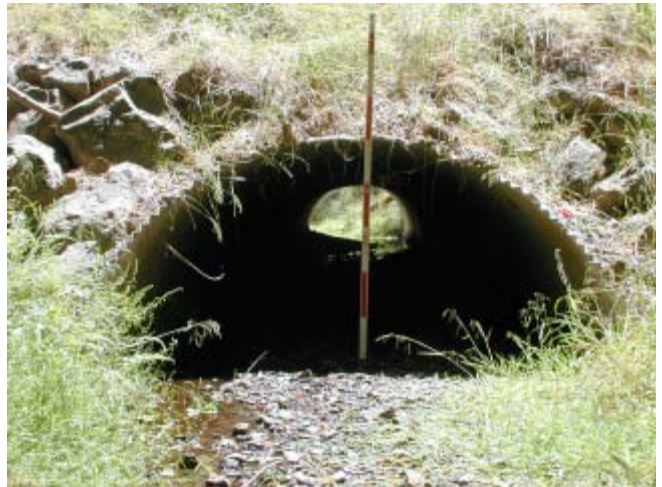
Getty's Creek 7/14/03 Looking upstream at culvert outlet.
