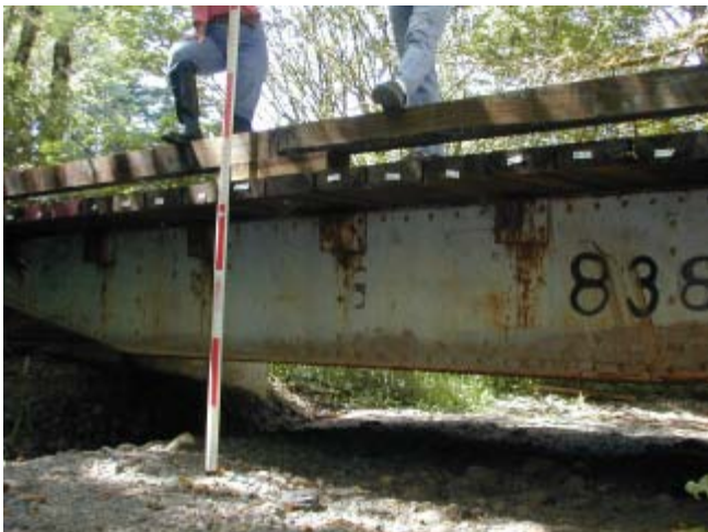
Swanson Creek 7/10/03 Looking downstream at bridge.
