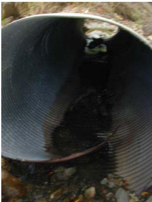
Feliz Creek Watershed 5/29/03 Looking downstream at culvert inlet.
