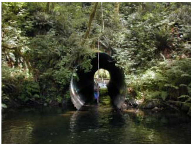
East Creek 7/15/03 Looking upstream at culvert outlet.
