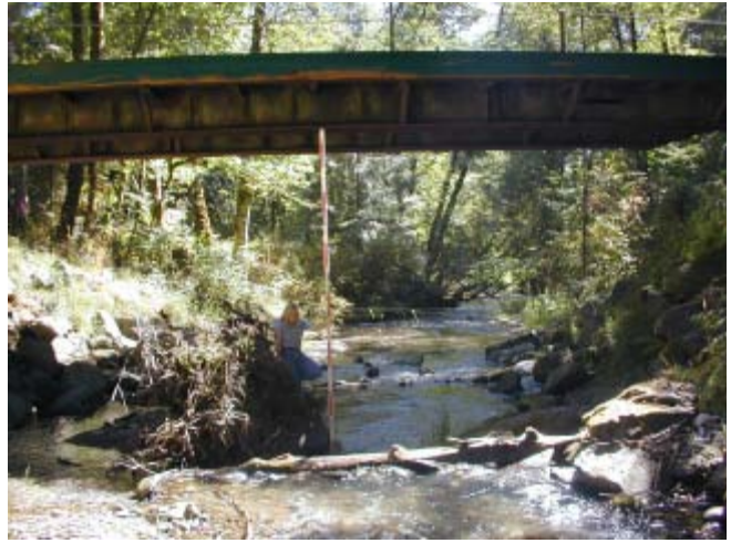
Alder Creek 8/18/03 Looking downstream at bridge.
