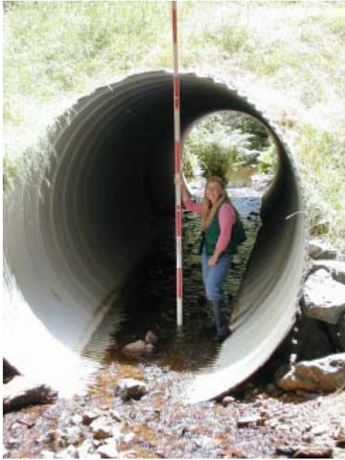
Hubbard Creek 7/10/03 Looking downstream at culvert inlet.
