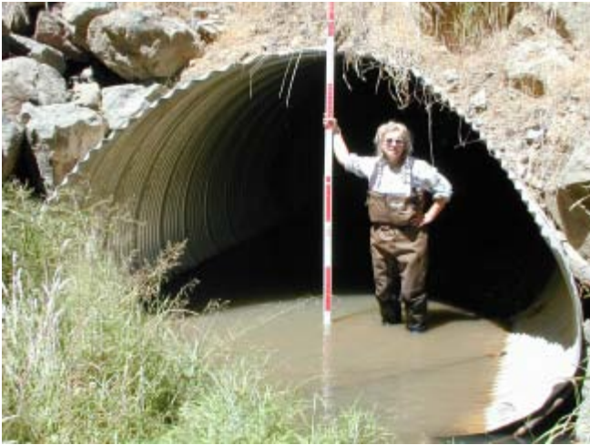
Getty's Creek 7/14/03 Looking downstream at culvert inlet.
