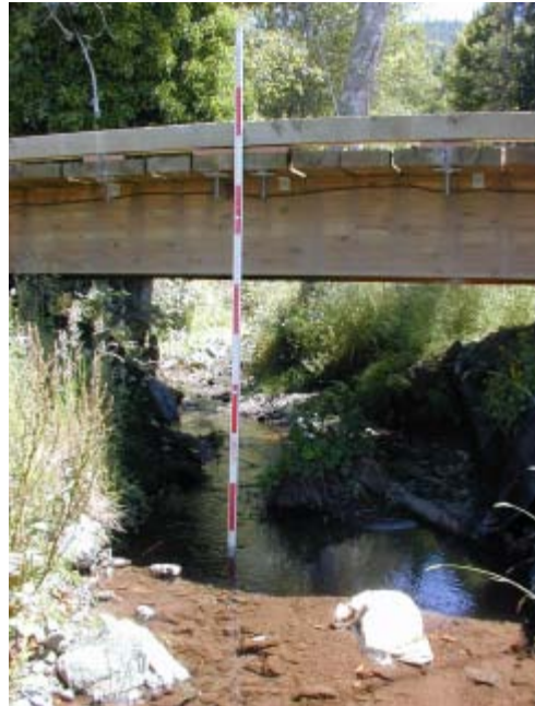
Turner Creek 7/10/03 Looking upstream at bridge.
