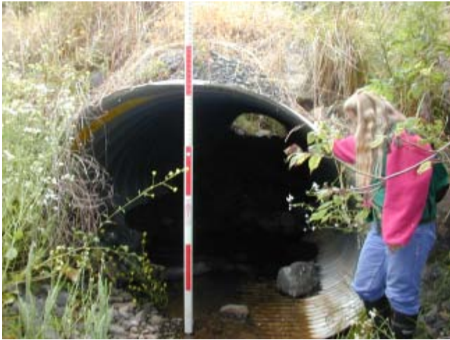
Edson Creek 7/10/03 Looking upstream at culvert outlet.
