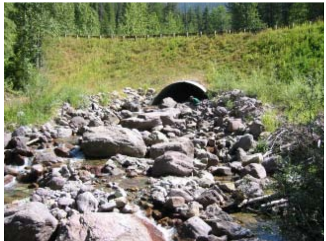
Riverside Creek 8/25/03 Looking upstream at culvert outlet.
