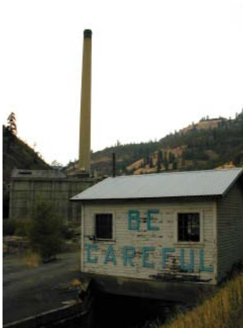
Snyder Creek 9/ 3/03 Old oil house over creek with stack in background.
