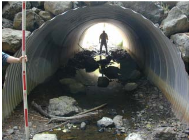
Green Creek 9/ 2/03 Looking downstream at culvert inlet.
