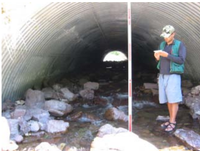
Felix Creek 8/25/03 Looking upstream inside culvert.
