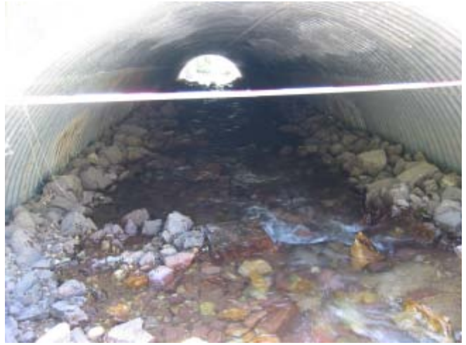
Harris Creek 8/25/03 Looking downstream inside culvert.
