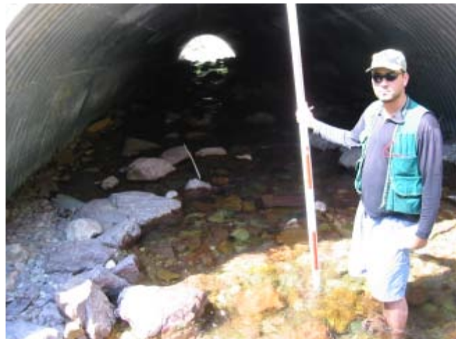
Felix Creek 8/25/03 Looking downstream at culvert inlet.
