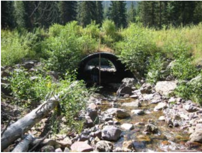
Margaret Creek 8/25/03 Looking downstream at culvert inlet.
