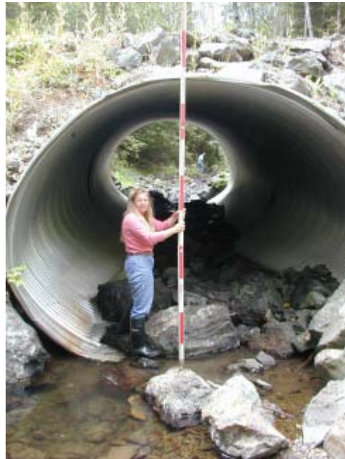
Indian Creek 7/10/03 Looking upstream at culvert outlet.
