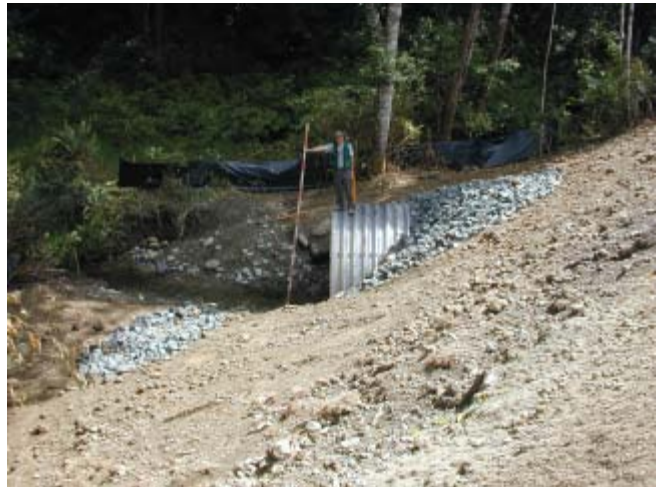
Tarboo Creek 8/12/03 Looking at culvert inlet from top of road fill.
