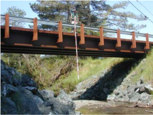
McCready Gulch 6/ 1/03 Looking downstream at bridge site.
