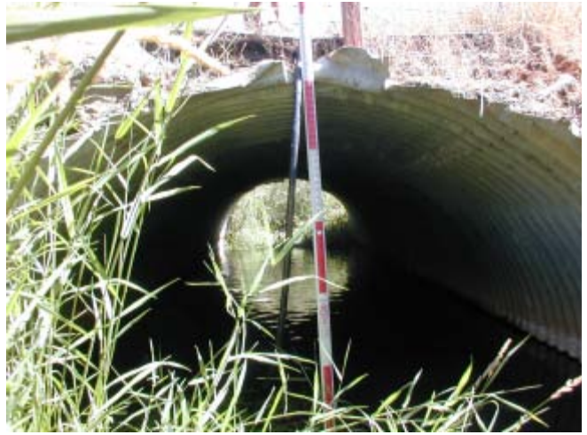
Wimer Creek 7/14/03 Looking downstream at culvert inlet.
