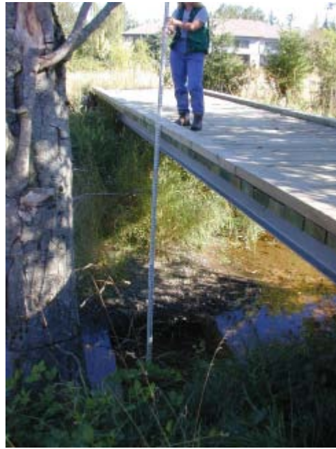
Squalicum Creek 8/18/03 MaryLou White at new bridge.
