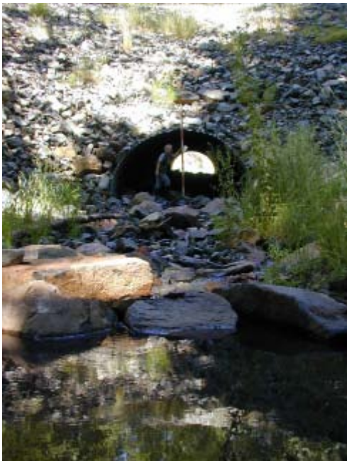
Finn Creek 7/ 9/03 Looking upstream at culvert outlet.
