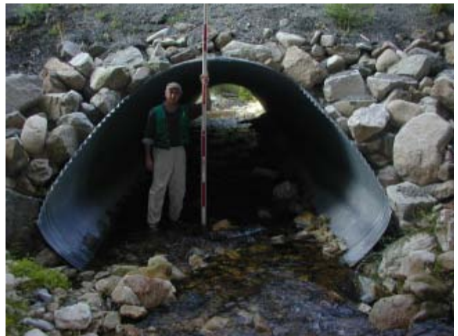
Wendover Creek 8/24/03 Looking downstream at the culvert inlet.
