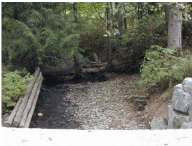
North Fork Newaukum Creek 8/11/03 Looking upstream from the upper culvert.
