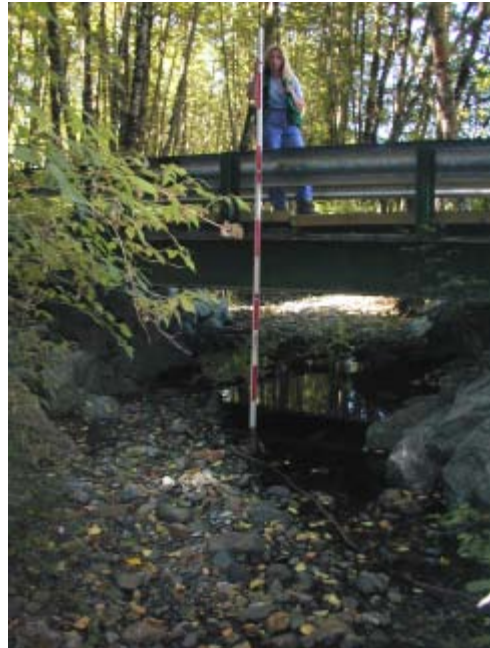
Klahoya Creek 8/18/03 Looking downstream at bridge site.
