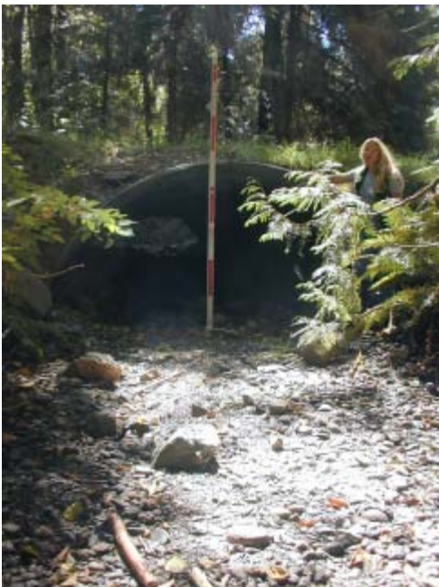
Klahoya Creek 8/18/03 Looking upstream at culvert.
