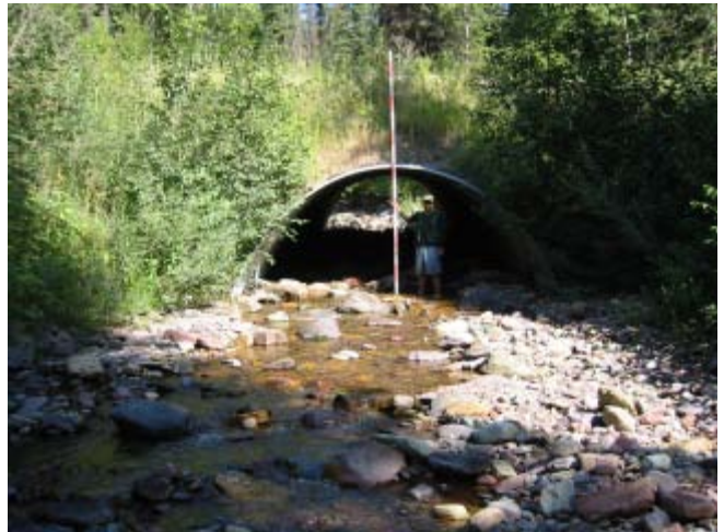
Margaret Creek 8/25/03 Looking upstream at culvert outlet.
