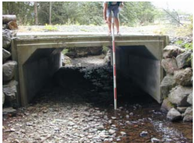
North Fork Newaukum Creek 8/11/03 Looking upstream at box culvert.
