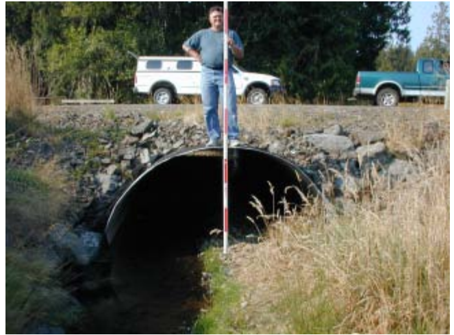
Bear Creek 9/ 2/03 Looking downstream at culvert inlet.
