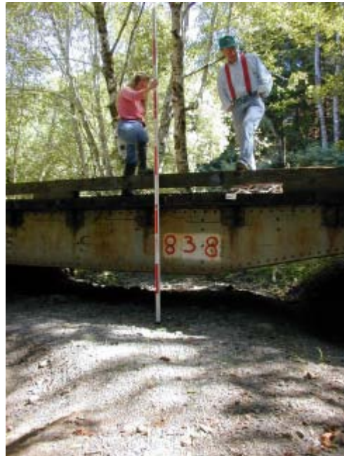
Swanson Creek 7/10/03 Looking upstream at bridge w/MaryLou White and Harry Hoogesteger.
