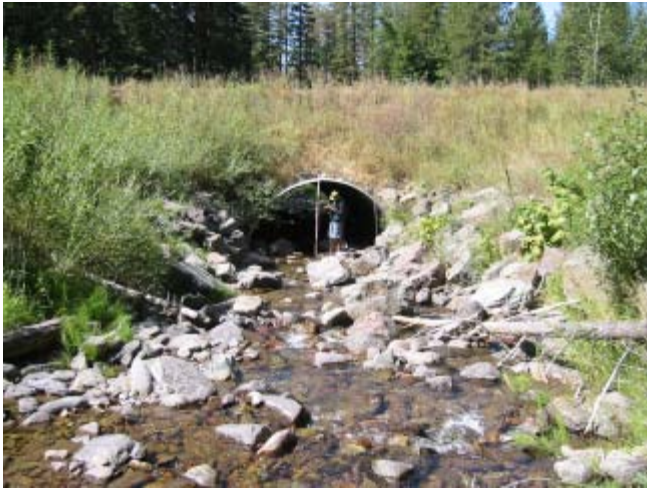
Murray Creek 8/25/03 Looking downstream at culvert inlet.
