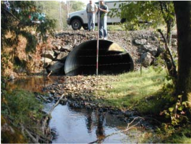
Bear Creek 9/ 2/03 Looking upstream at culvert outlet.
