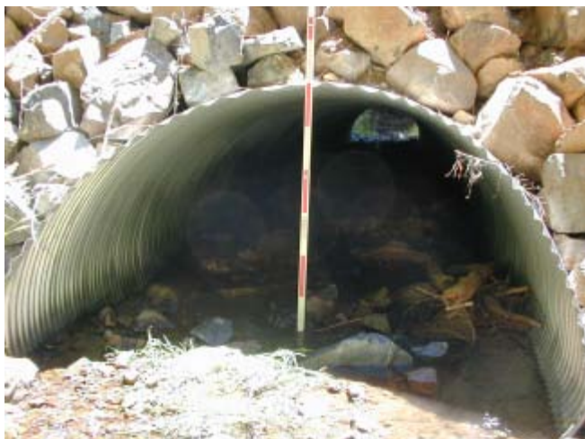
Finn Creek 7/9/03 Looking downstream at the culvert inlet.
