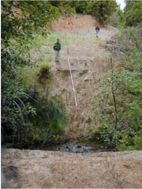
Little North Fork Navarro 5/30/03 Culvert removal site and associated decommissioned road.
