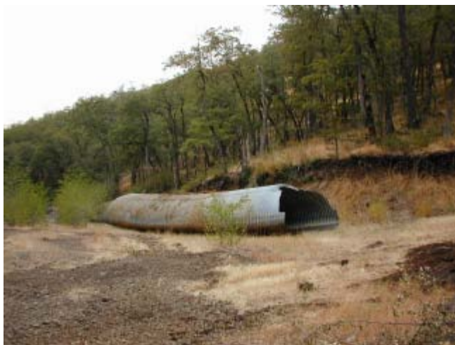
Snyder Creek 9/ 3/03 Old pipe that was removed for bridge installation.
