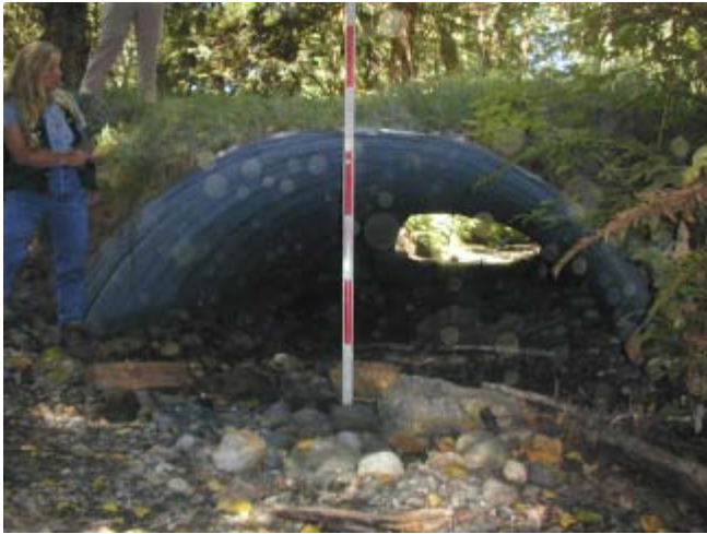
Klahoya Creek 8/18/03 Looking downstream at culvert, downstream-most site.
