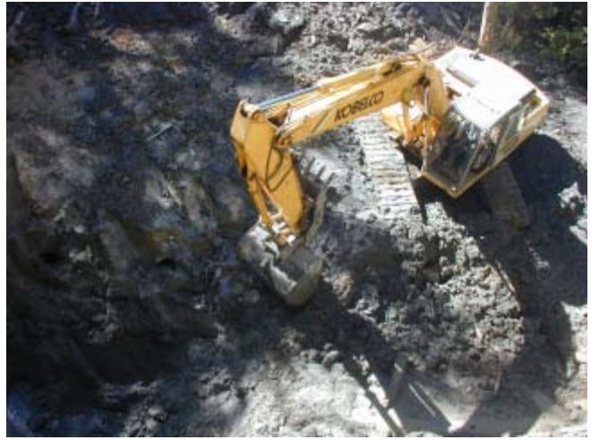
Shoeshel Creek 8/18/03 Hydraulic excavator culvert construction.
