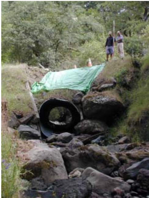
Feliz Creek Watershed 5/29/03 Looking upstream at culvert replacement site.
