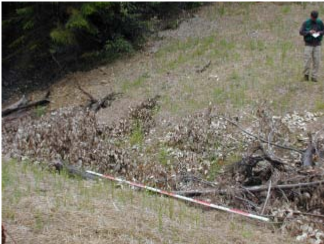
Little North Fork Navarro 5/30/03 Dry channel stream crossing on a decommissioned road.
