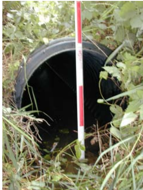
Little Easy Creek 7/13/03 Looking downstream at culvert.
