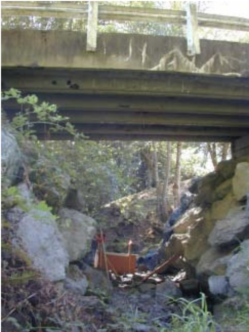
Red Creek 8/18/03 Looking downstream at bridge.
