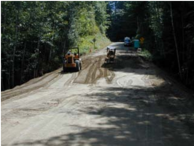
Tarboo Creek 8/12/03 Grading the road above the Tarboo installation.
