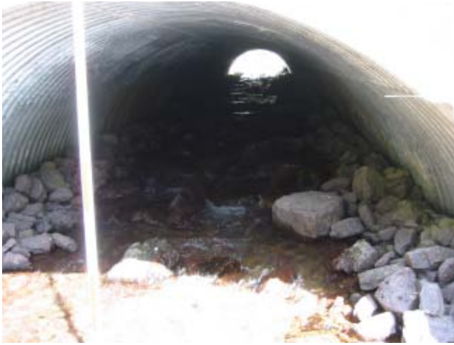
Harris Creek 8/25/03 Looking upstream inside culvert.
