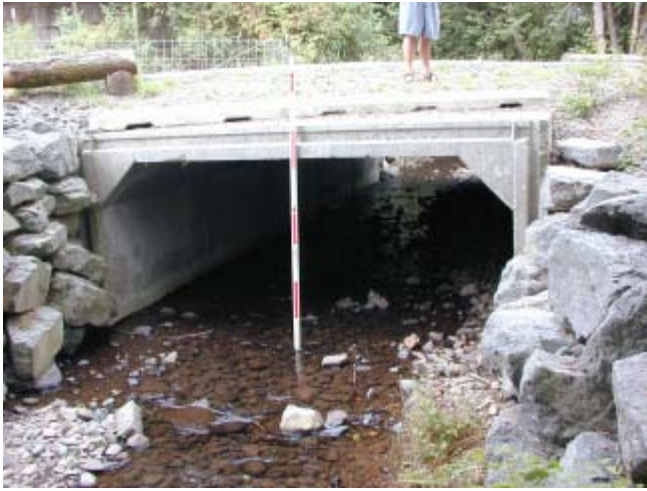
North Fork Newaukum Creek 8/11/03 Looking downstream at box culvert.
