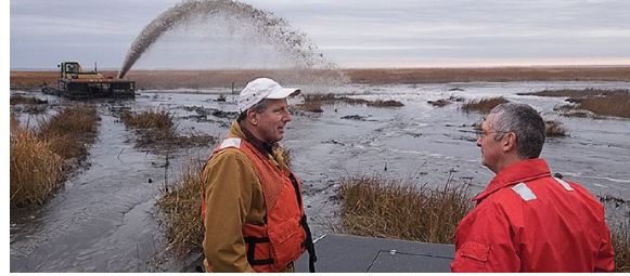
Thin-layer dredge is applied to Blackwater NWR.
