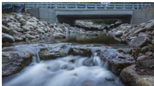
Culvert restoration in North Elba, NY. Source: TNC.
