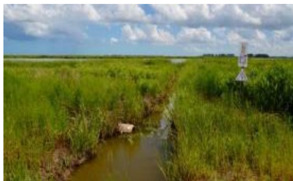
A small channel dug on Prime Hook NWR to reconnect the flow of water (Cape Gazette).
