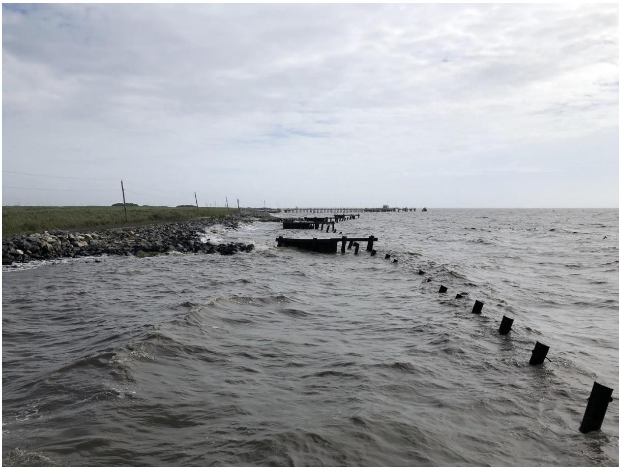
**Figure CS1-1.** Area of former marsh and beach that is now open water with large “dilapidated bulkhead/rip-rap” structure installed to protect Port Mahon Road. During storms, water overtops the rocks and inundates the road.
