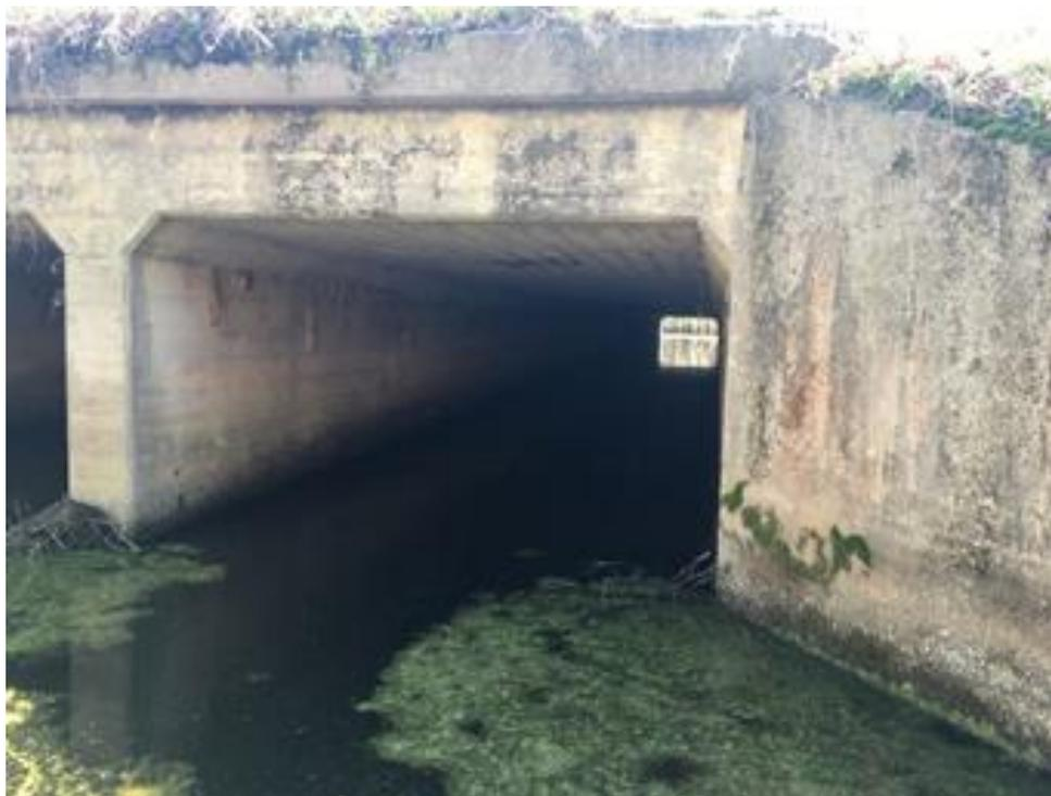
**Figure CS1-1.** Example of a box culvert that would be assessed as part of a regional analysis looking at fish passage barriers across the state.
