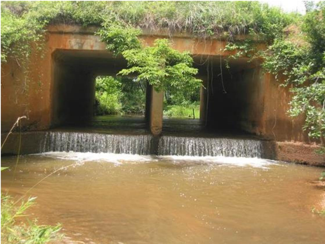
**Figure CS2-2. Perched double barrel box culvert showing a plunge pool and stream widening immediately downstream of the structure. Dawson County, GA (USFWS photo).**
