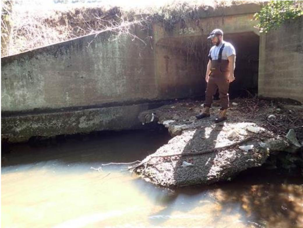
**Figure CS2-1.** Example of a box culvert that would be assessed as part of a regional analysis looking at fish passage barriers across the study area. Credit: US Fish and Wildlife Service.
