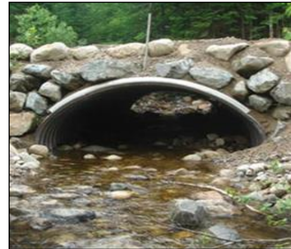
Culvert after replacement. Credit California Fish Passage Forum
