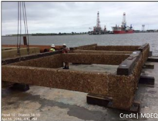
Above, concrete panel structures that will be used to construct artificial reefs.
