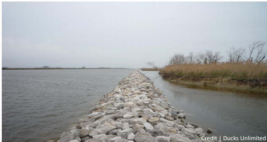
The construction of this breakwater structure will protect the Candy Abshier Wildlife Management Area as well as creating valuable coastal salt-marsh habitat.
