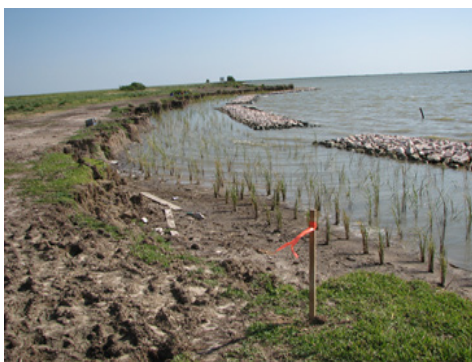
This project completed the engineering and design for a project that will protect up to 6,000 linear feet of shoreline and approximately 30 acres of coastal marsh habitat in West Galveston Bay.
