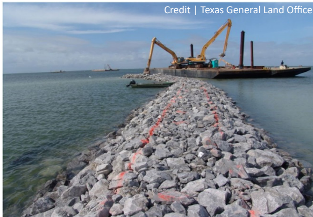
Rock breakwaters, similar to the above photo, will be constructed to protect critical habitat on and around Galveston Island State Park.
