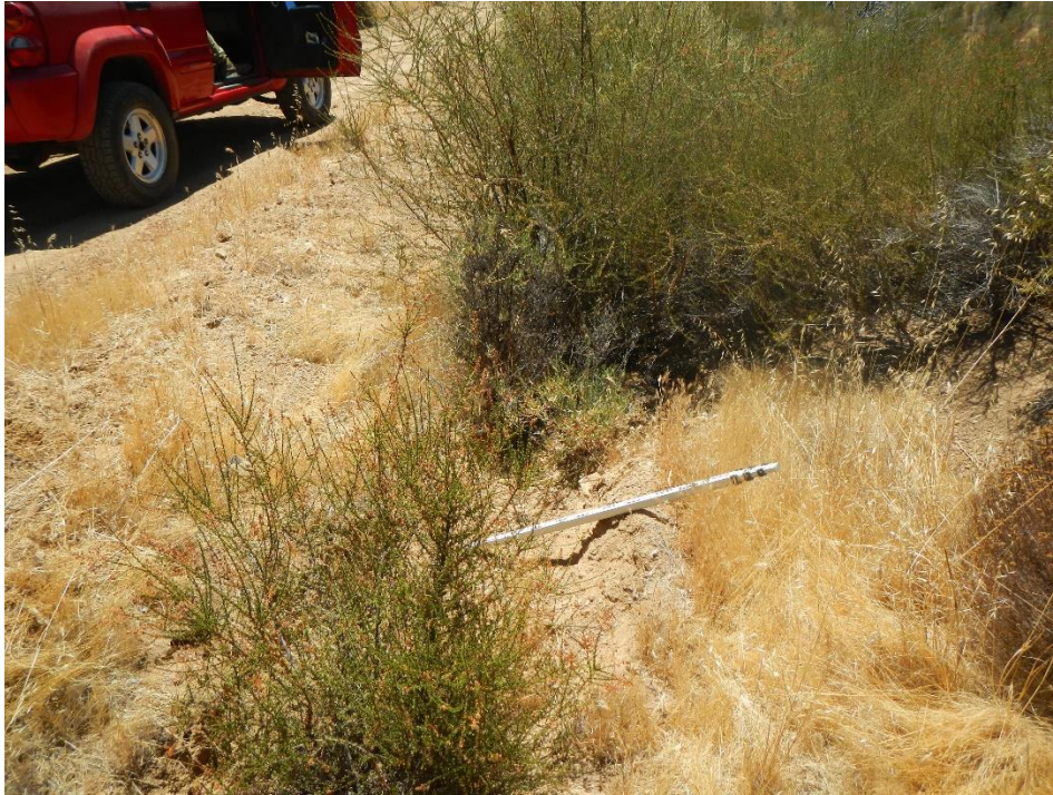
Photo 3 – Gullied lead off ditch on 9N11.4
