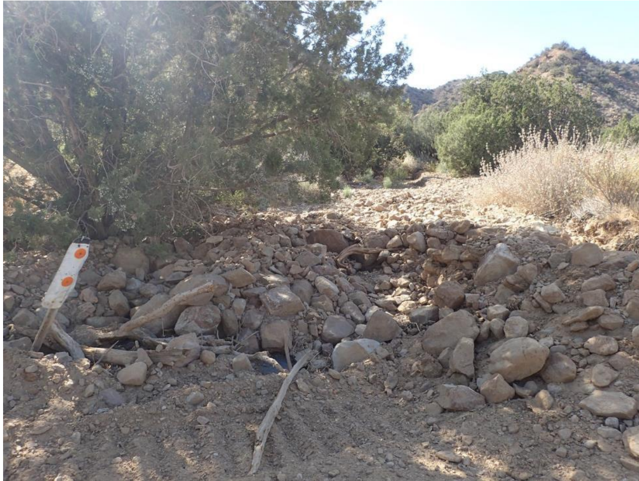
Photo 16 – Culvert stream crossing blocked by debris flow on 9N11.2
