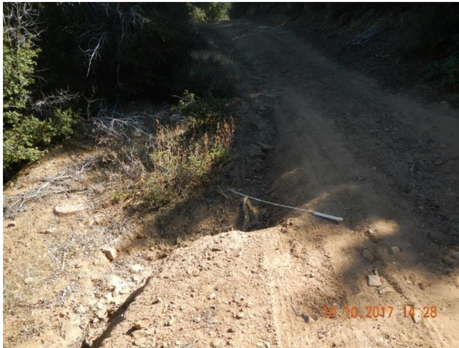
Photo 8 – Erosion associated with non-engineered drain point on 9N11.4
