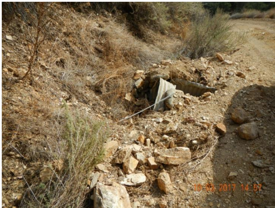
Photo 5 – Buried ditch relief culvert on 11N04.3
