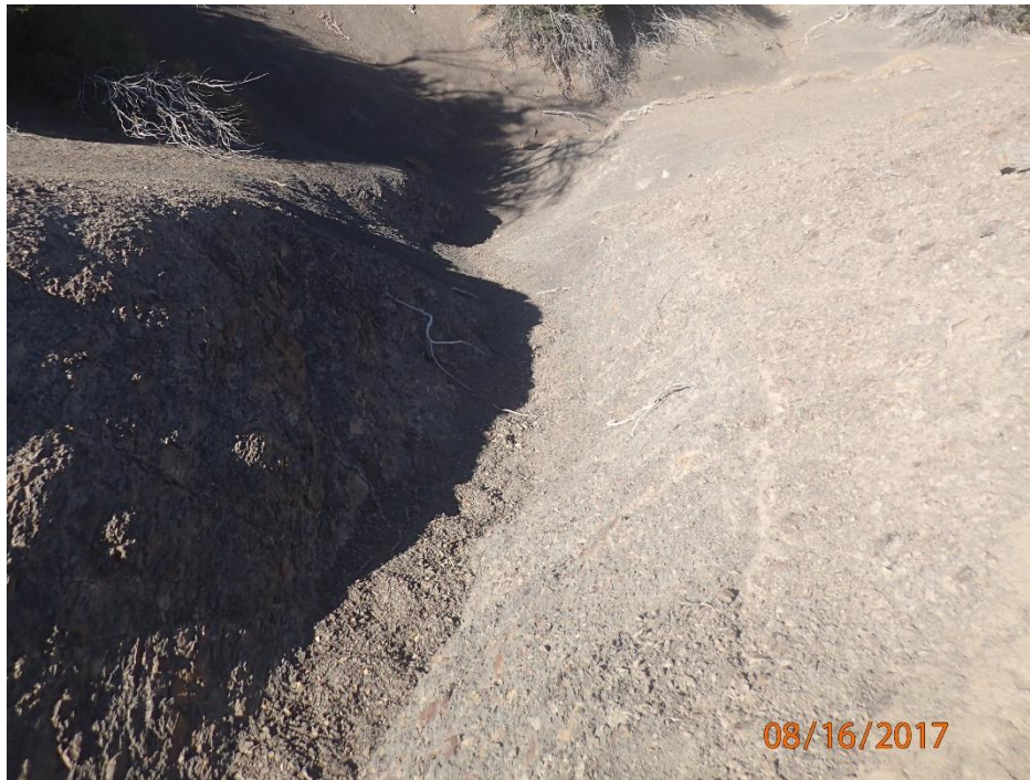
Photo 3 – Gullied lead off ditch on 9N11.4
