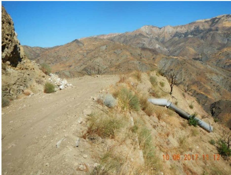
Photo 5 – Buried ditch relief culvert on 11N04.3
