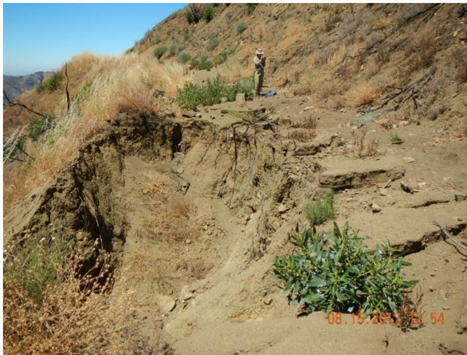
Photo 8 – Erosion associated with non-engineered drain point on 9N11.4
