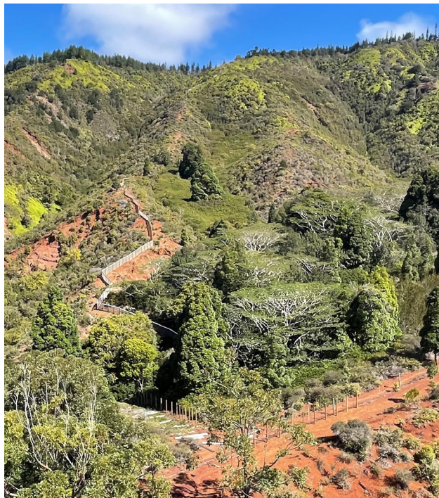
Predator-proof fence under construction
