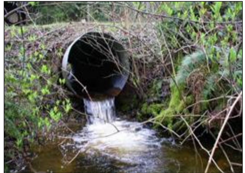
Perched culvert. Credit California Fish Passage Forum
