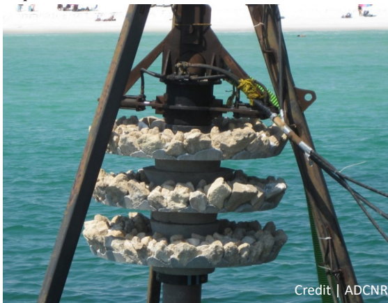
Above, juvenile fish shelters attached to a fiberglass pile that will be embedded in a concrete slab and lowered to the seabed.
