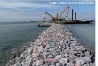
Rock breakwaters, similar to the above photo, will be constructed to protect critical habitat on and around Galveston Island State Park.
