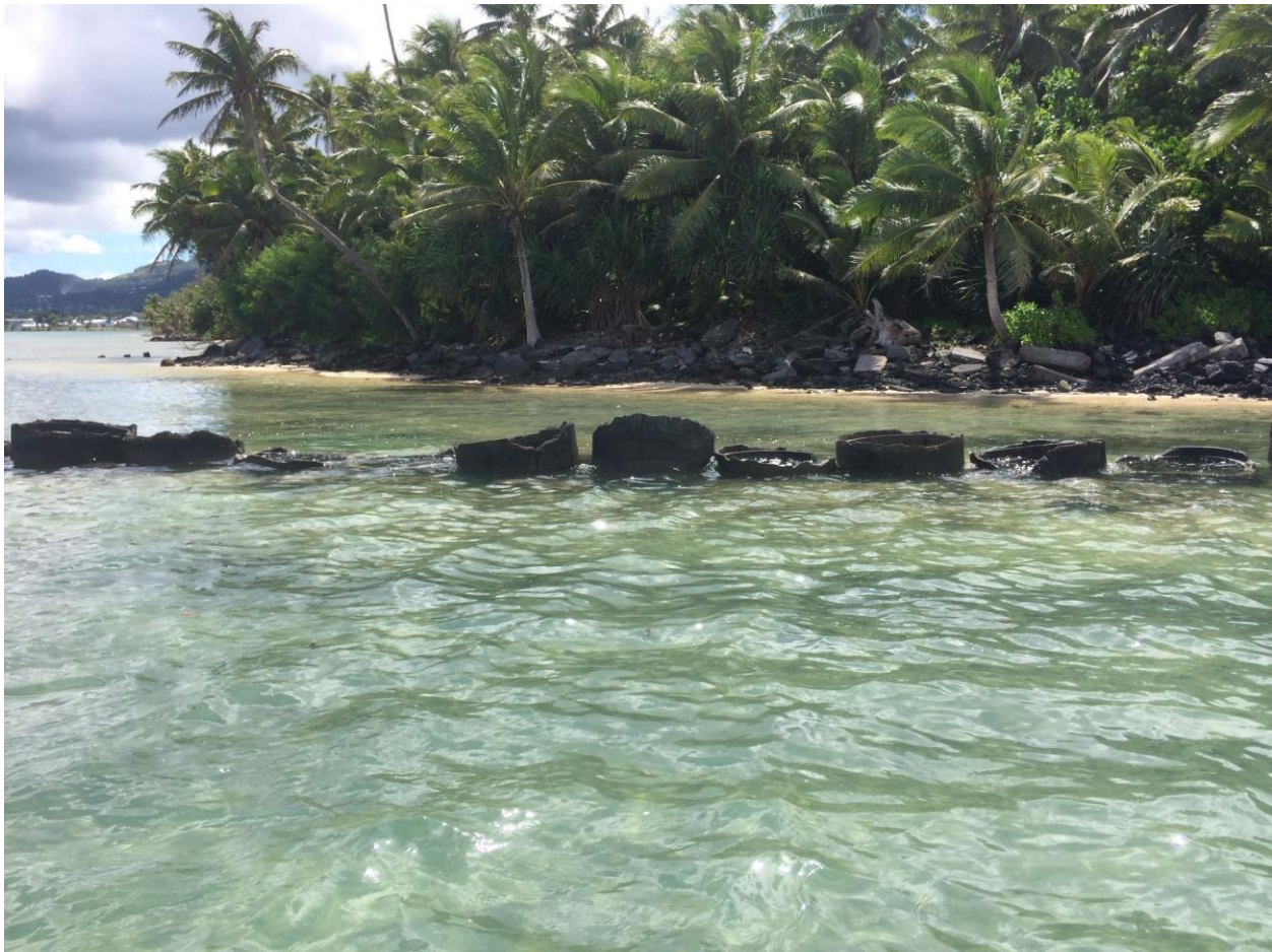
Figure 28. View of the Nu'uuli Uta living shoreline design site. Shoreline erosion is visible along the shore. Prior to the 2009 earthquake and ongoing subsidence, this site featured several feet of dry sand that has since been inundated. Photo credit: Kelley Anderson Tagarino, University of Hawai'i at Mānoa.
