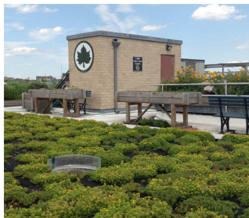
The fund supports development of infrastructure such as this green roof at a New York City park.
