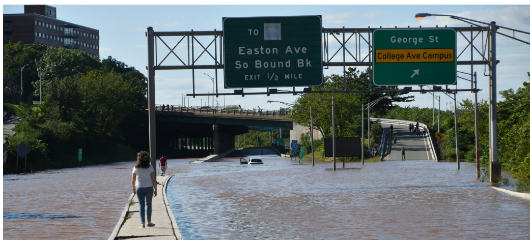
Flooding in New Jersey after Hurricane Ida
