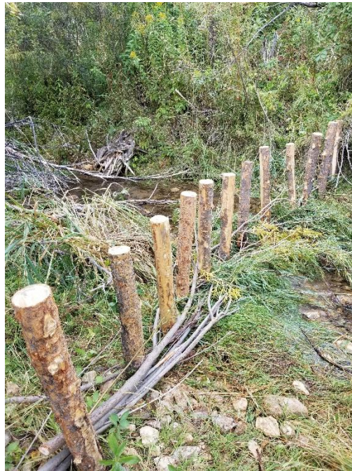
Completed Beaver Dam Analog project
