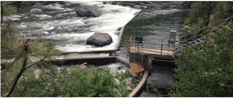
Before photo of the Cascade Orchard Irrigation Company transaction, which includes the large diversion structure that served as the largest passage barrier on Icicle Creek. After photo showed restored flows and removed diversion.
