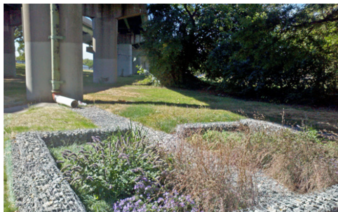
Figure 1: Finished highway overpass landscape detention system in Flushing Meadows-Corona Park
