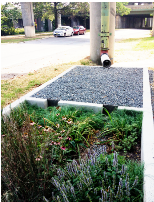
Figure 9: Flushing Bay HOLD SYSTEM™ (finished basin 1)
