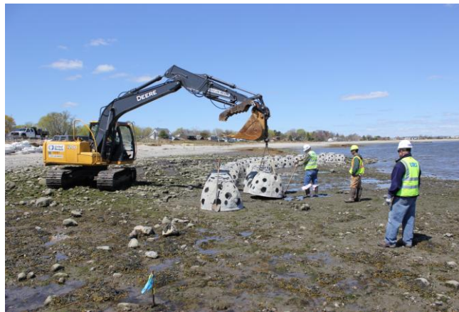
Figure 2. Installation of Reef Balls
