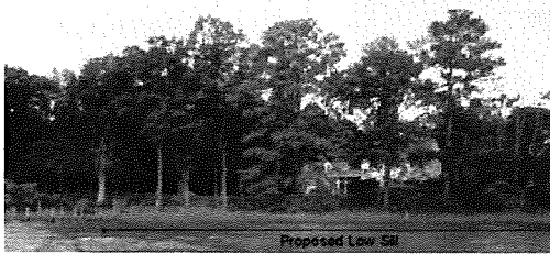
Pons Point facing southeast Transitional bank face erosive base of bank with existing marsh fringe
