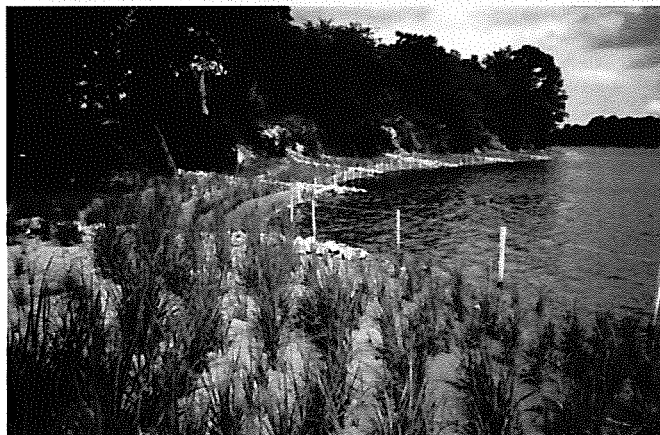
Marsh grass plantings with sand fill and short, stone groins 3 months after installation on Wye Island, Kent County.
