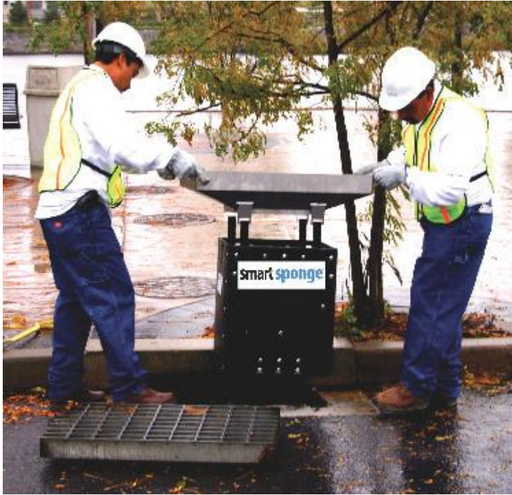
The lightweight Drop In series of the Ultra Urban Filter installed as part of the Norwalk Filter Project, Government Engineering 2006, p. 17.
