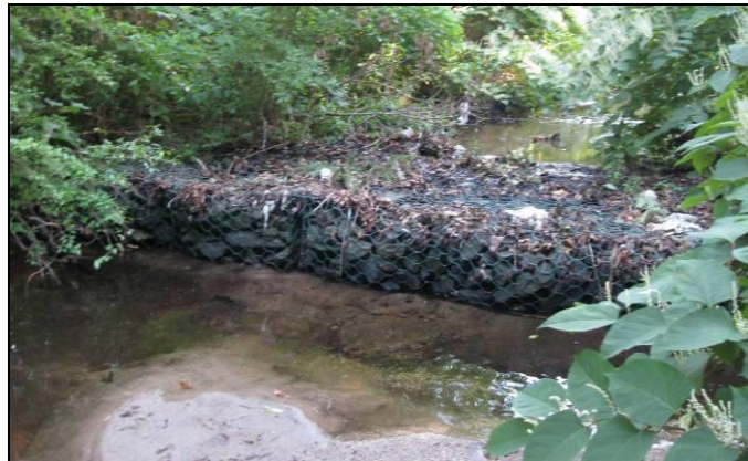
Gabion wall along reach CSB-04
