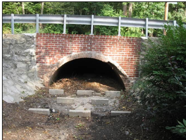
This arched culvert, OT-01, discharges to the box culvert that conveys Cold Spring Brook beneath Harbor Road.
