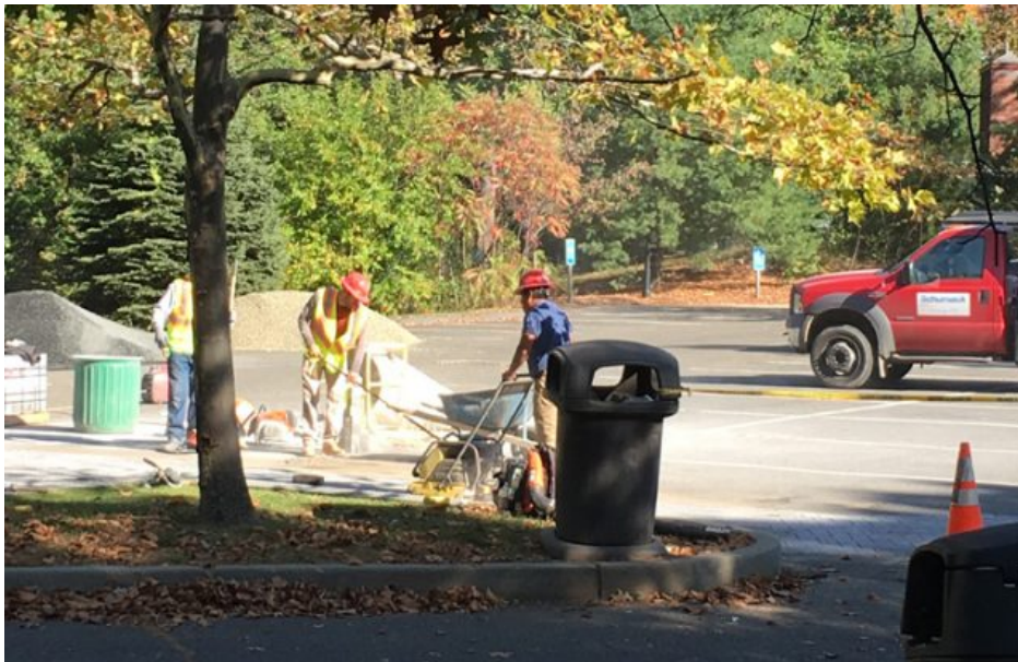
More permeable pavers were installed in the Zoo's parking lot.
