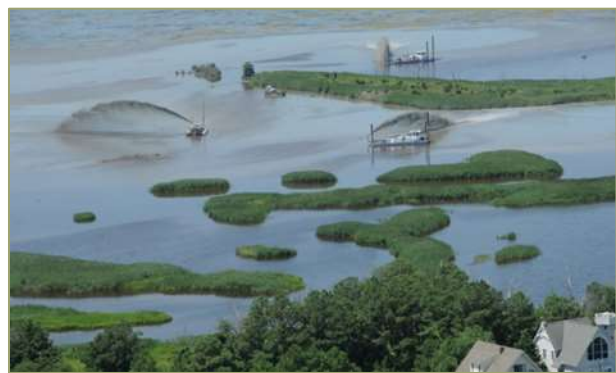
Dredge work to drain flooded marsh at Prime Hook National Wildlife Refuge (Richard Weiner)
