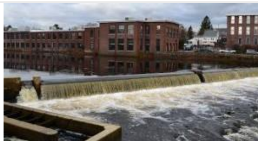
Ipswich Mills Dam, funded for a removal feasibility study, is scheduled to be removed in summer 2019. Source: Ipswich River Watershed Association.
