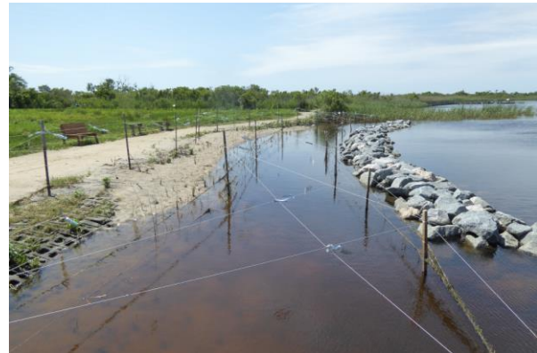
Back Bay National Wildlife Refuge completed living shoreline construction (project final report).
