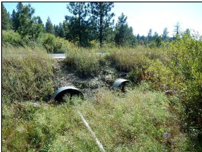
6.3 Looking southwest over culverts under Estate Drive. Most of upslope study area drains through these culverts. Photo date 8-11-15
