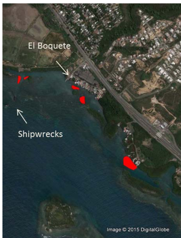
Figure 8. Additional boating impacts near El Boquete, Peñuelas, PR.
