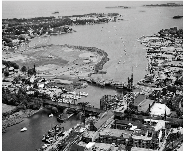
Aerial view of Norwalk Harbor in June 1987. Photo: US Army Corps of Engineers.
