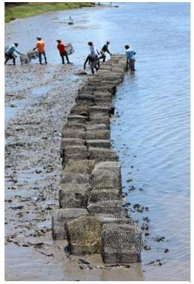
Figure CS2-1. Crab Traps to Oyster Reefs Project. Shellfish Research Section of South Carolina Department of Natural Resources building a crab trap reef with the help of Clemson University student volunteers (site is at South Fenwick Island, SC).
