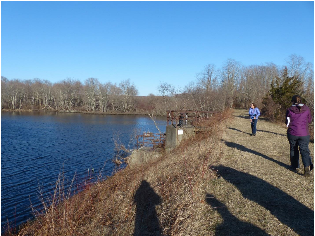
Figure CS2-1. Earthen dam and impoundment of the Kickemuit River.
