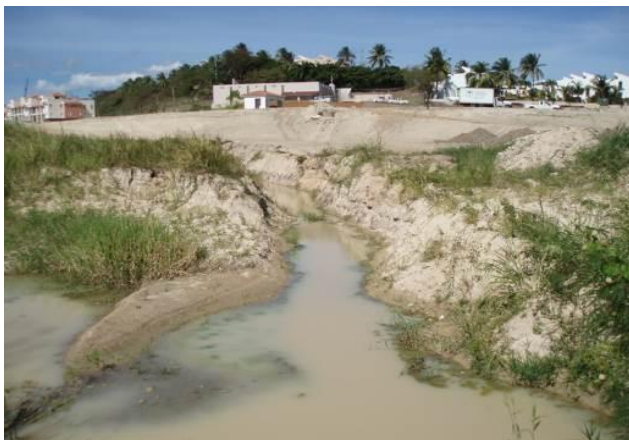
Evaluate construction sites, quarries, or other areas where erosion control measures should be used to prevent offsite turbid discharges.
