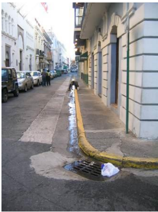
Look for washwater, dumpster juice, automotive products, or other discharges entering the drainage system from residential and commercial areas during dry weather. Identify what the behaviors are that need to be targeted for education to reduce these sources of pollution.
