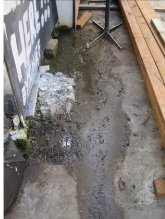
Look for washwater, dumpster juice, automotive products, or other discharges entering the drainage system from residential and commercial areas during dry weather. Identify what the behaviors are that need to be targeted for education to reduce these sources of pollution.
